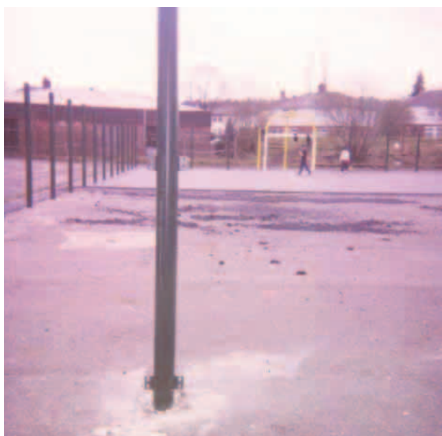
Figure 30 New basketball court being built on the Ashy, Allison Blythe, March 2008
