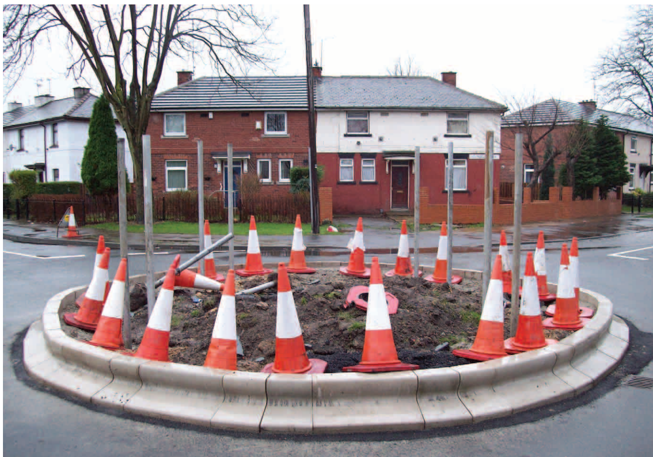
Figure 27 Scholemoor roundabout, E.-J. Milne, December 2007
