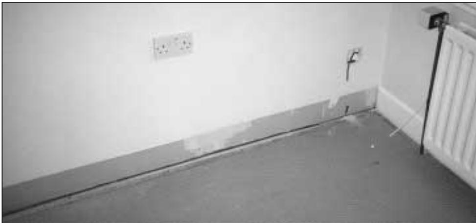
It became evident that installing cabling would be more difficult than expected, in spite of provision of cableways behind skirting boards and under door thresholds. The dwelling had been fitted out as a show flat and gripper rods used to fit carpets prevented skirting boards from being easily removed. In addition, routing of the radiator pipework hindered the use of intended cableways. As well as hindering the initial installation this was also likely to cause difficulties in future adaptation.
