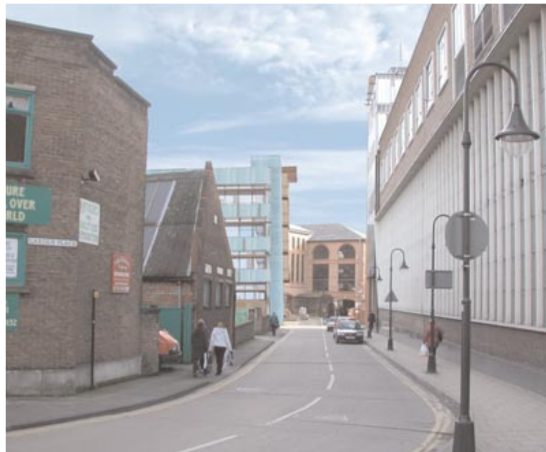
Panter Hudspith's winning proposal as seen from Garden Place © Panter Hudspith Architects
