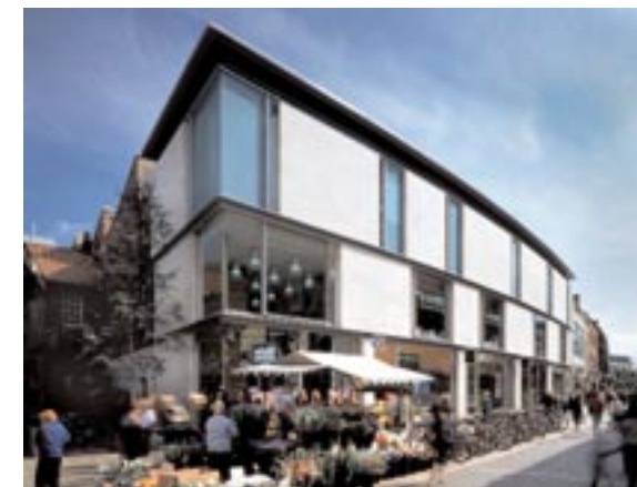
1-3 Daveygate, Panter Hudspith Architects
