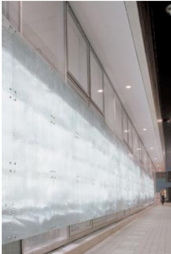
Slumped glass used at the “Floating Wall” at Yorkshire Artspace, Sheffield
