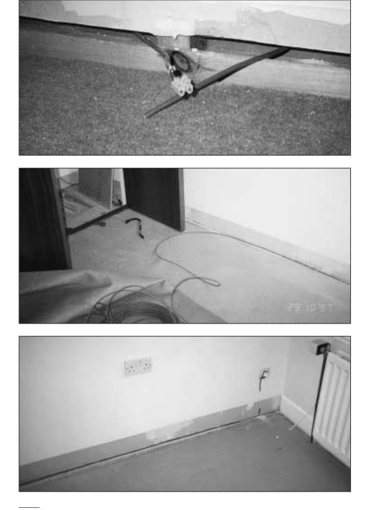
It became evident that installing cabling would be more difficult than expected, in spite of provision of cableways behind skirting boards and under door thresholds. The dwelling had been fitted out as a show flat and gripper rods used to fit carpets prevented skirting boards from being easily removed. In addition, routing of the radiator pipework hindered the use of intended cableways. As well as hindering the initial installation this was also likely to cause difficulties in future adaptation.
