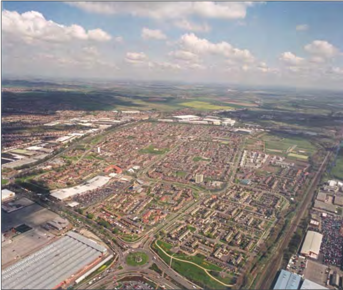
An aerial shot of a regenerated Castle Vale. The work was carried out by Castle Vale Housing Action Trust, certainly the best funded organisation in the JRF Programme
