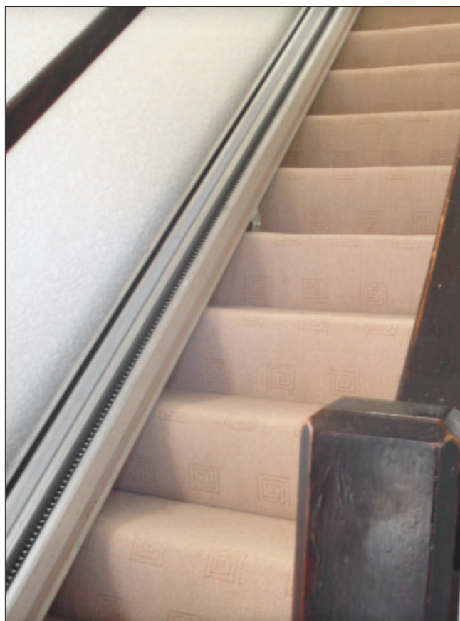
Image 8 Staircase with handrails on each side and a stairlift track
