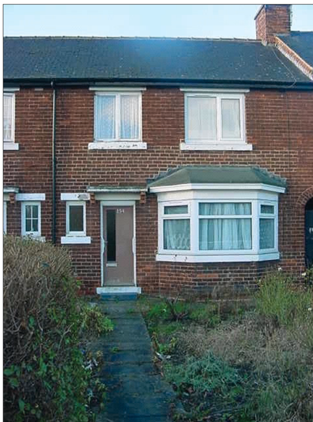
Image 1 A typical paved pathway leading to a stepped front-entrance door
