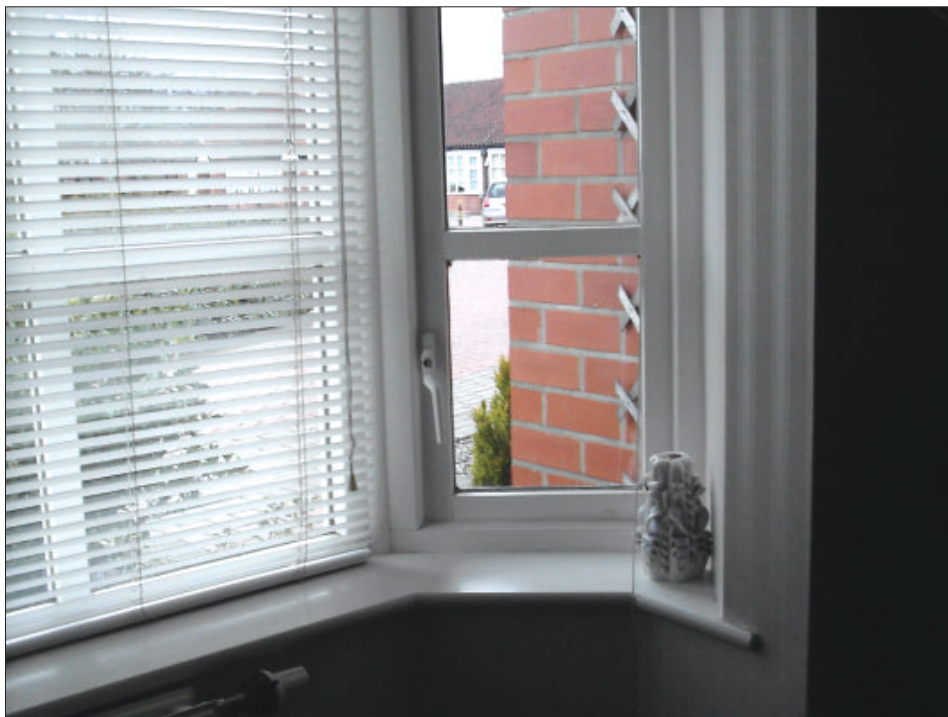
Image 6 Window with lower handle opening
